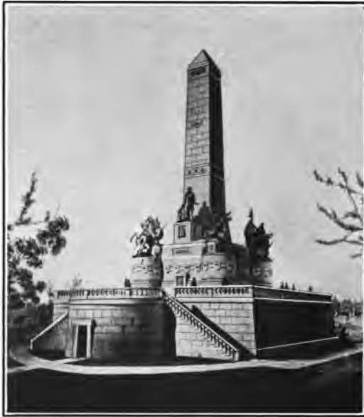
LINCOLN MONUMENT Springfield, Illinois, Larken G. Mead, Architect
